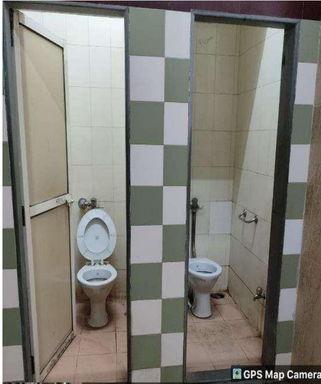
Washroom facility for Girl
